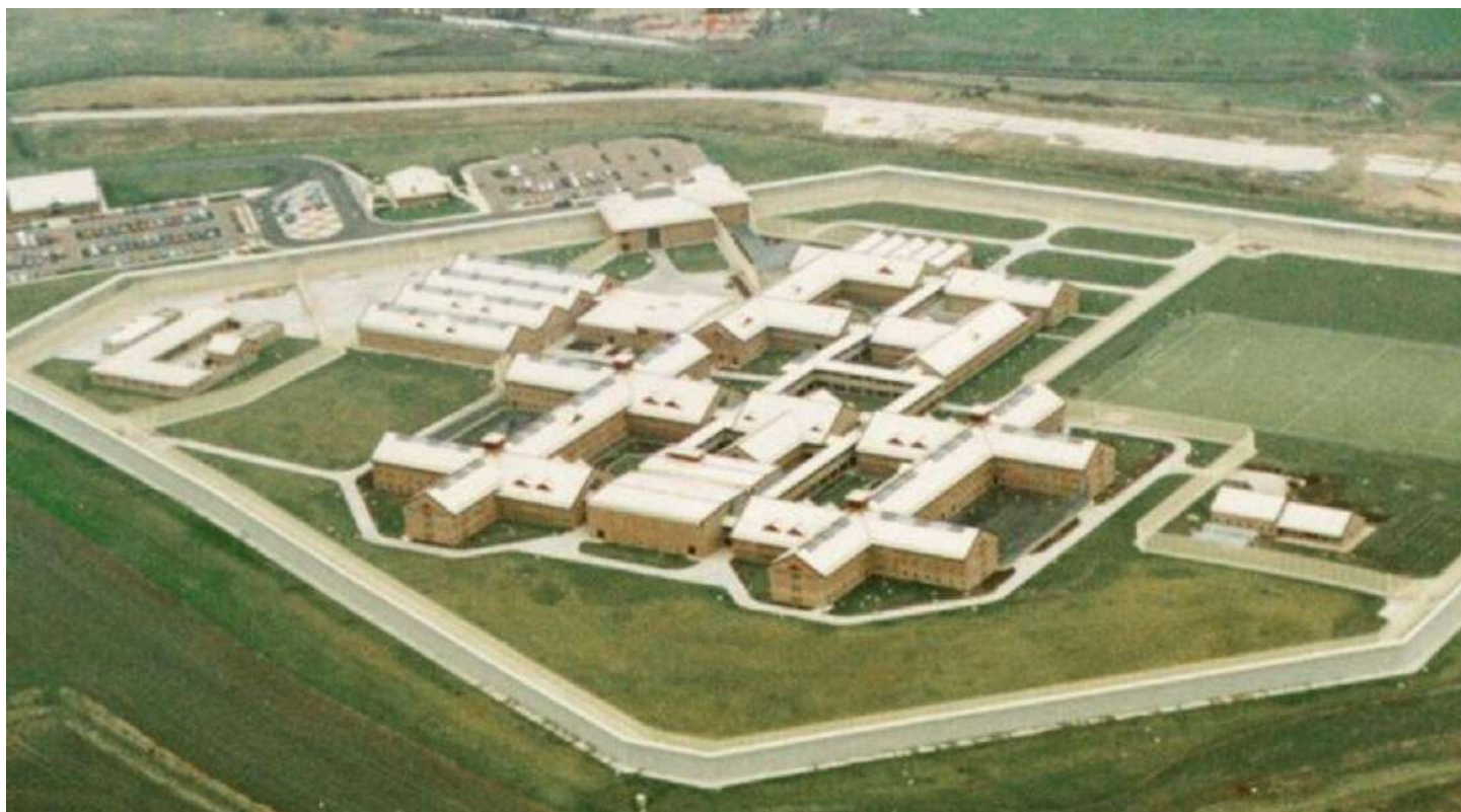
Figure 9 HMP Holme House
